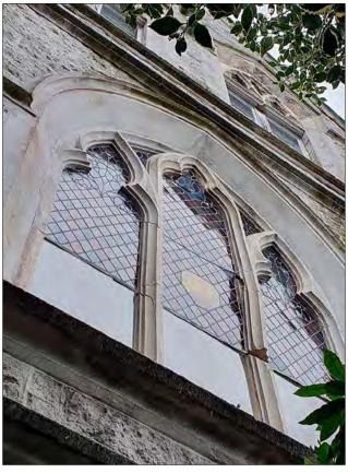
The window in place, with one of the mullions broken and cracked, and no longer supporting the weight bearing down from above.
